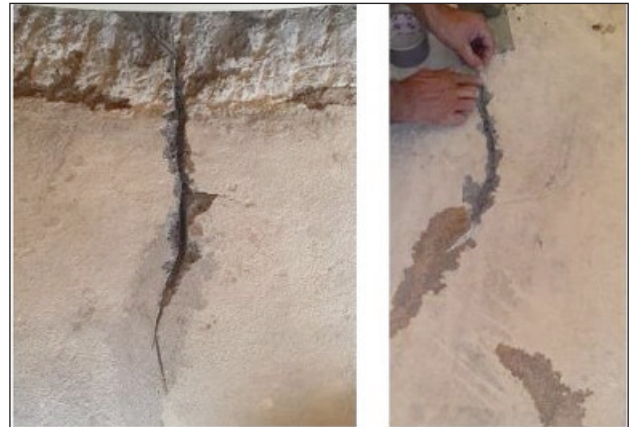
WTG 1 – Repair process
